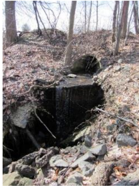
Outlet Destabilization
