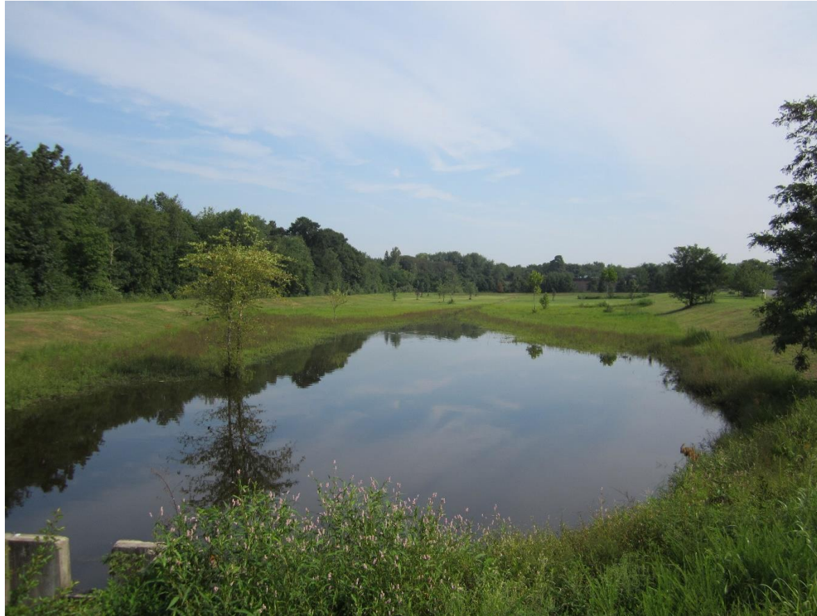
Standing water in detention basin
