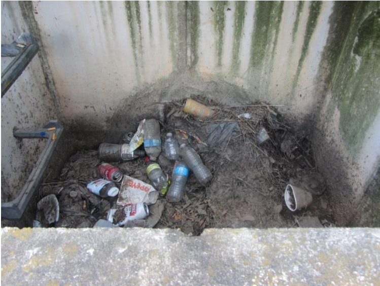
Accumulation of floatables from outfall
